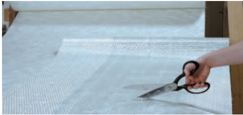
1. Fiberglass material is cut to size.
