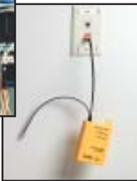
Locate LAN cable at the patch panel
