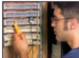
Easily identify telephone and LAN pairs.
