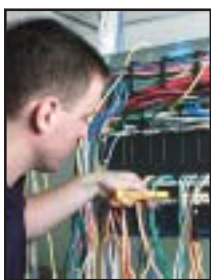
Locate LAN cable at the patch panel
